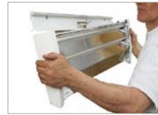
Hinge the luminaire to the wall bracket.
