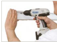
Fix the bracket to the wall using screws.
